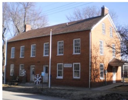
1851 Carpenter and Paint Shop
